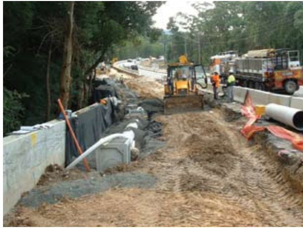
Central Coast Highway, upgrade work.
