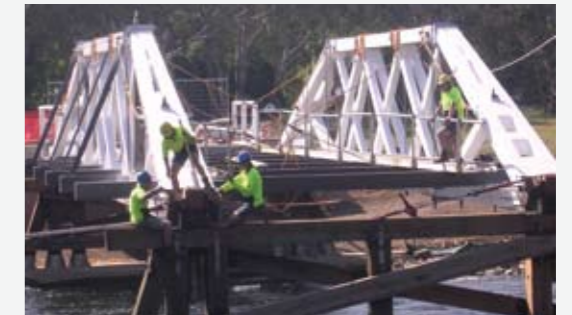
Restoration works on Junction Bridge, Tumut.
