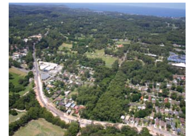
Aerial view of Central Coast Highway (Terrigal Drive to Carlton Road).
