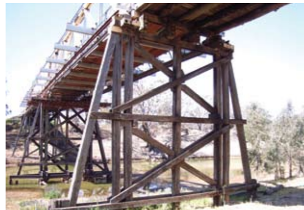
Coonamit Bridge, Wakool.
