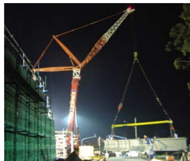
Night works: Erection of the bridge girders, June 2008.
