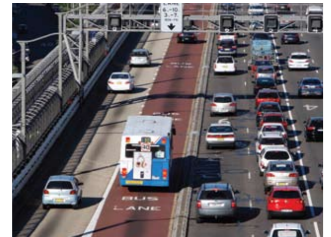
Sydney Harbour Bridge bus lane.
