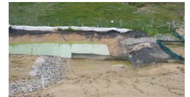
Sediment basin, Coopernook to Herons Creek upgrade.
