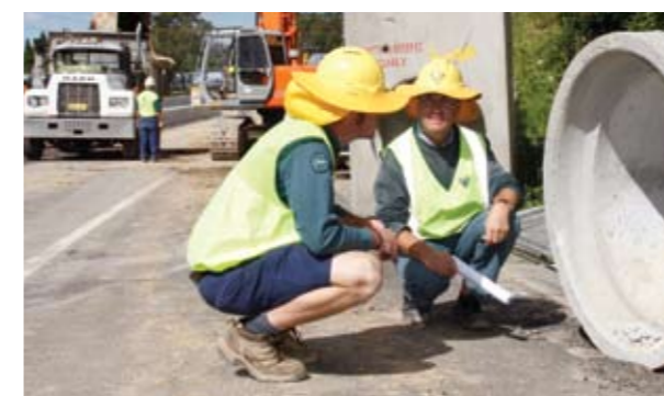
RTA staff carrying out an OHS inspection on site.
