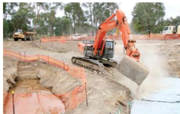
Work underway on the Southern Hume Highway Duplication
