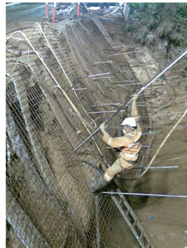
Maintenance engineer from Southern region repairing road damage at Bulli Pass.
